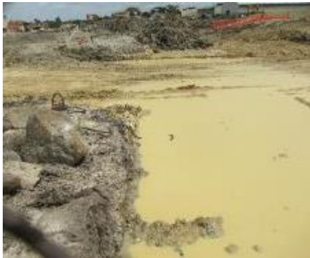
Poor site management results in sediment laden stormwater making its way into creeks impacting on riparian habitats.
